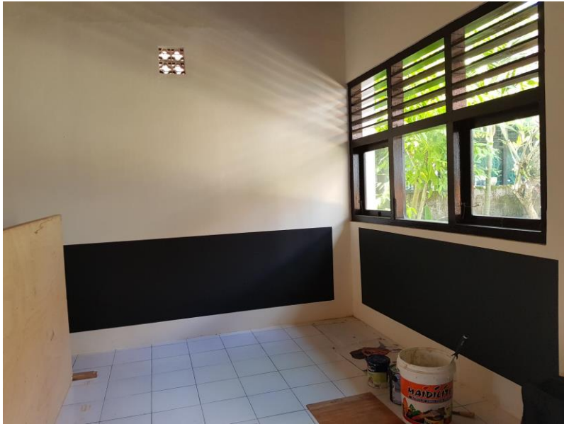
Chalkboard wall painting (on progress) start 14 Dec 2021)
